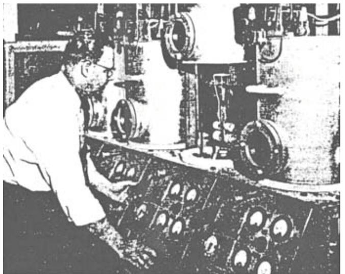
Looks as if he might be piloting a space ship, but actually Norman Berry is vacuum-sealing the tubes with this mechanism.
